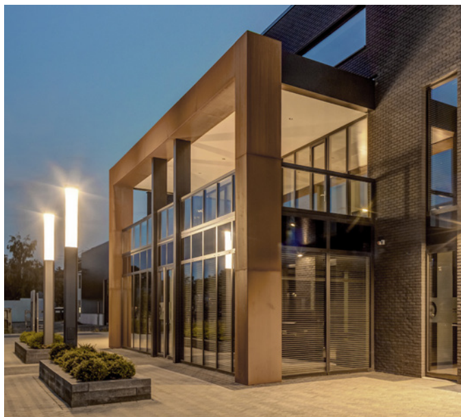
New building electrical wholesaler Robri - Wekerom - Netherlands
