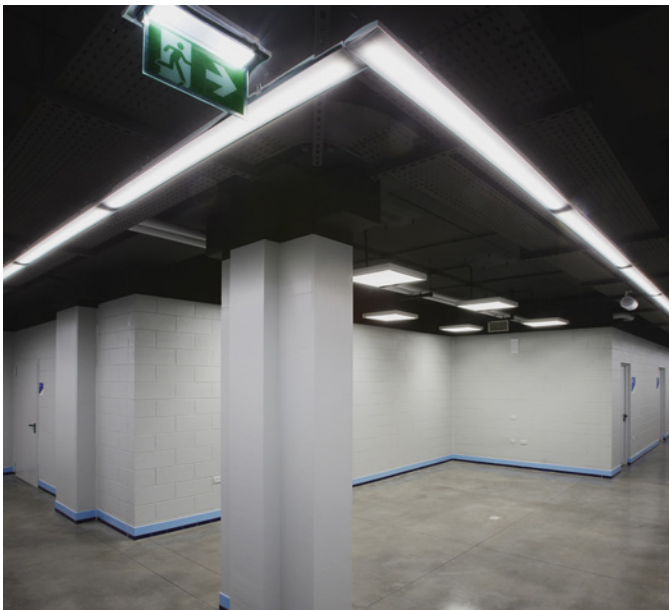
Albinoleffe stadium - Zanica - Italy
