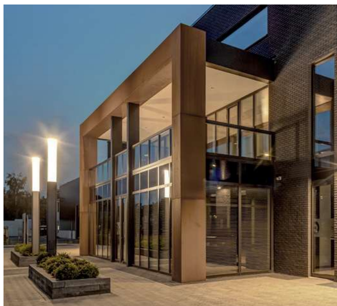
New building electrical wholesaler Robri - Wekerom - Netherlands
